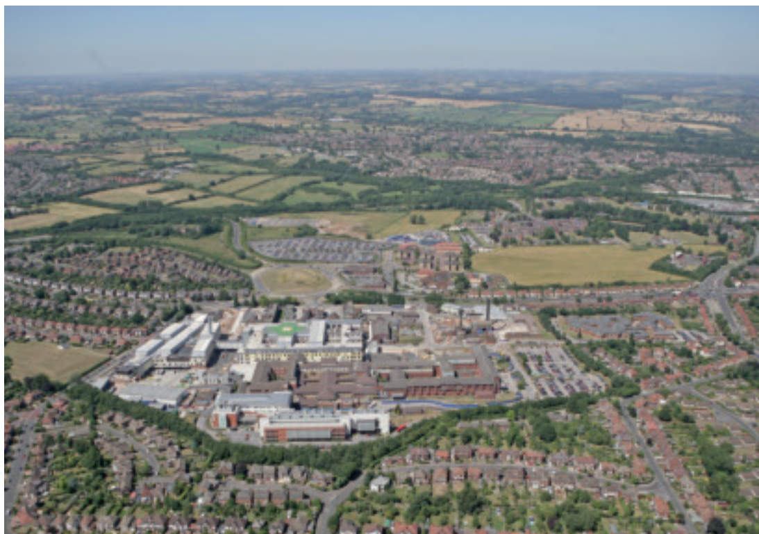
■ Aerial view of the Derby City General Hospital including Phase 1 of the new build - August 2006
