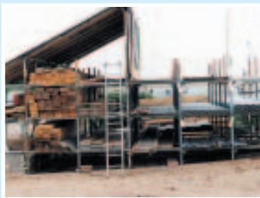
Good practice in materials storage
