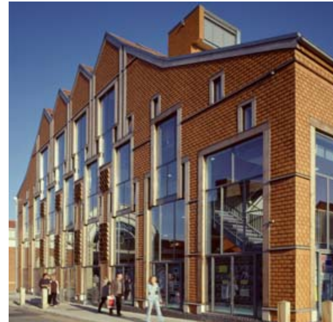
Lichfield Garrick project
