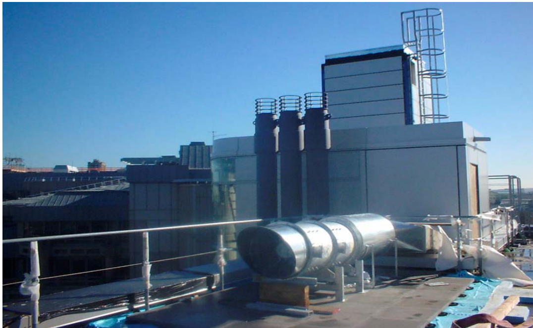
5/10/04 – Roof Level Ductwork Installation
