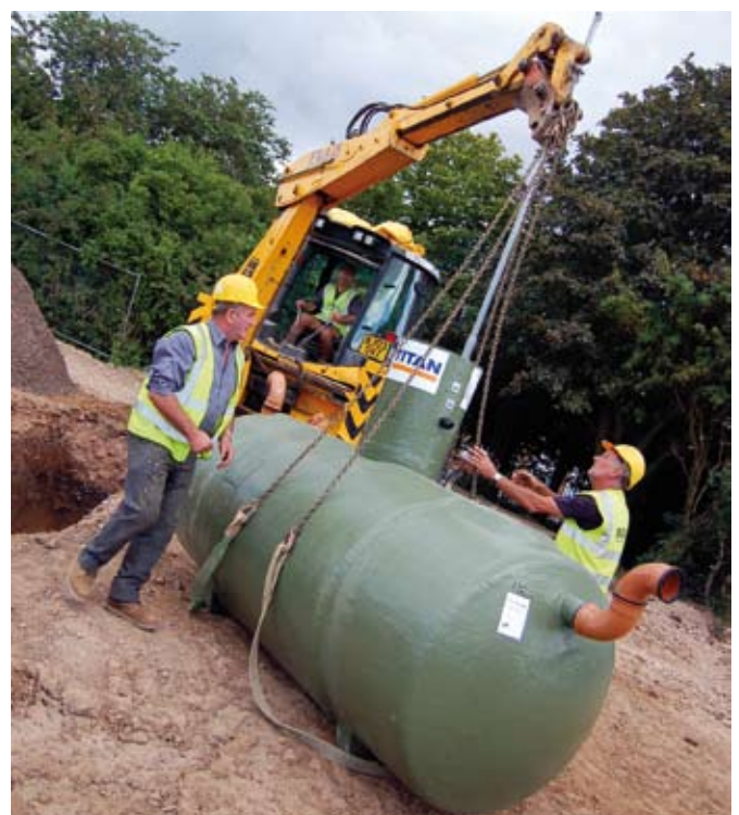
Installation of the rainwater harvesting tank
