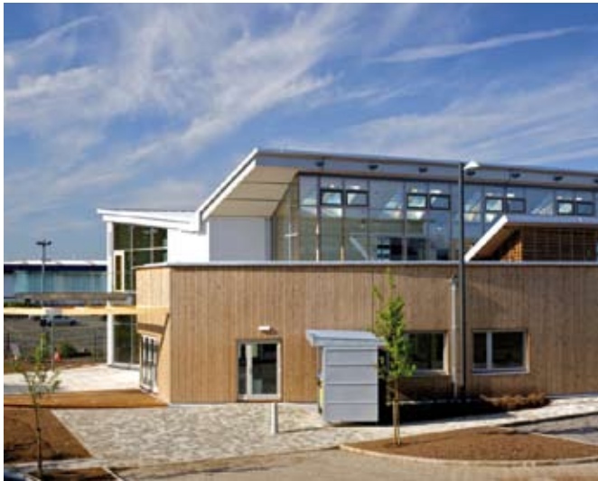
SBC completed in April 2008
