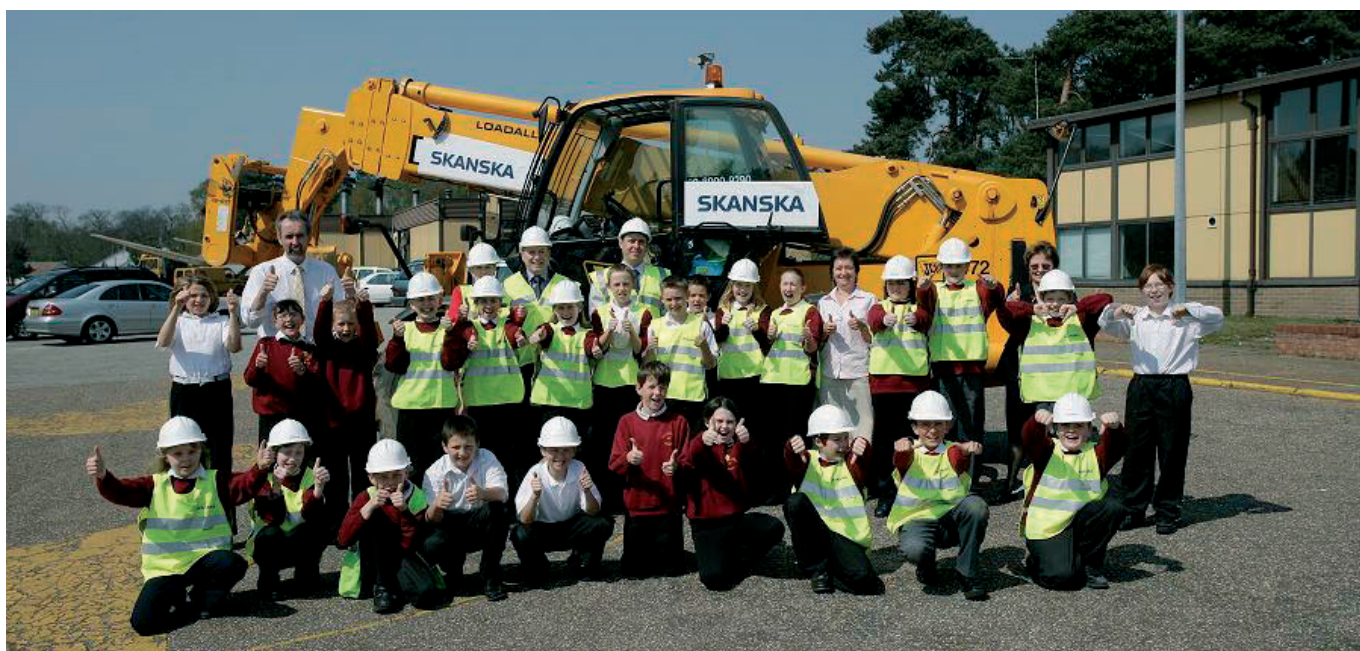
Some children from the local primary school were given a tour of the site
