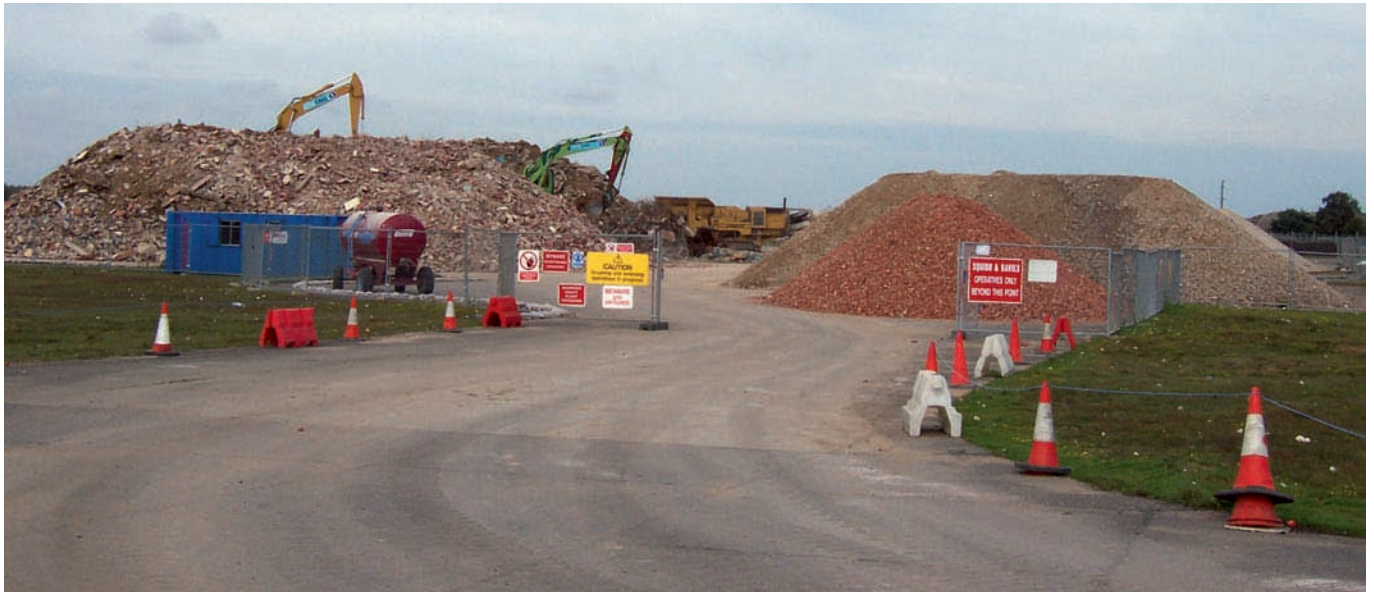
Segregated crush material
