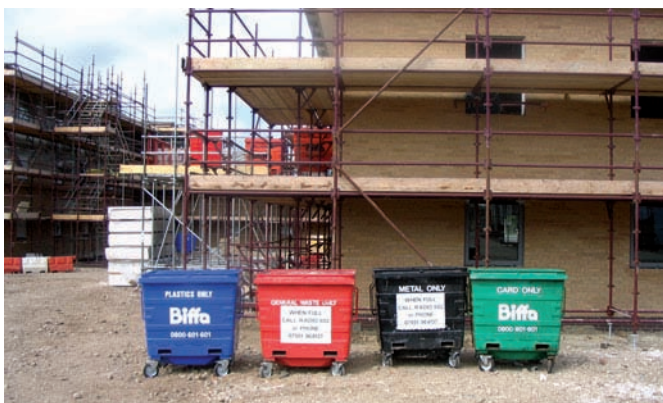
Waste was segregated into colour coded bins
