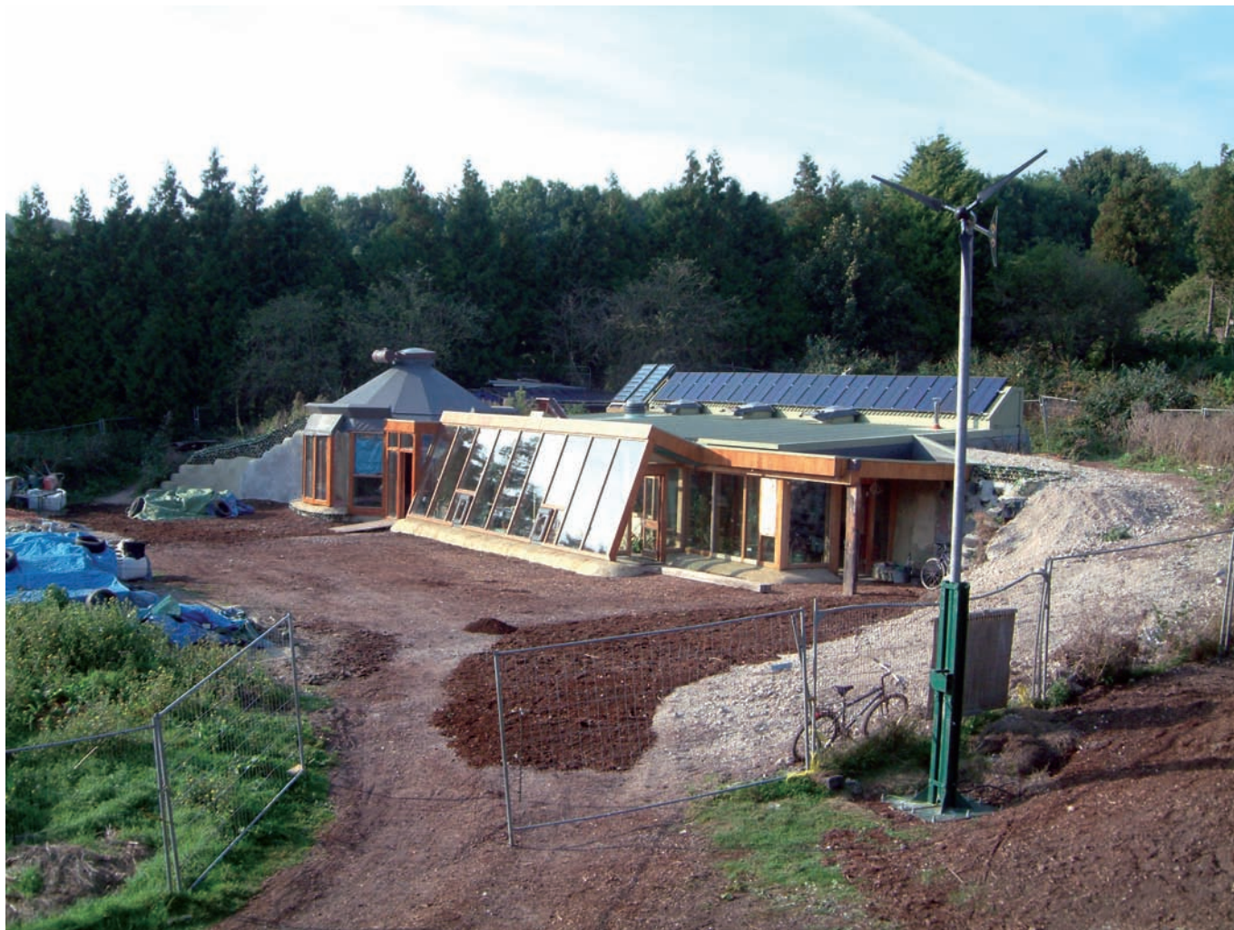
Earthship Brighton during construction
