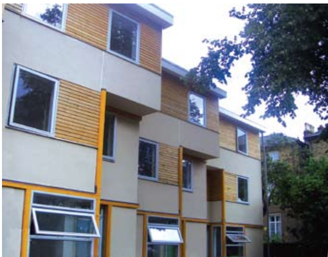
The houses vary from 4 to 7 person units. They are all designed to Lifetime Homes Standards
