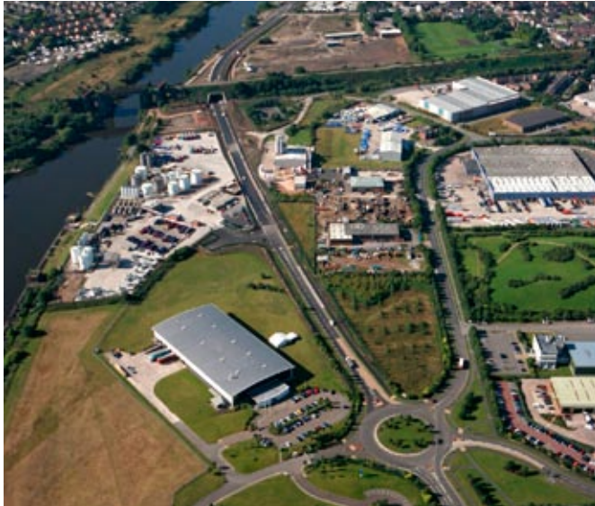
Aerial view of the completed road
