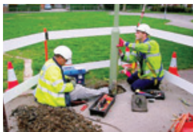
SEC street lighting engineers working to repair a column
