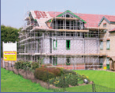
Works progressing on the Bentley Hotel
