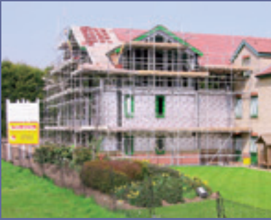
Works progressing on the Bentley Hotel
