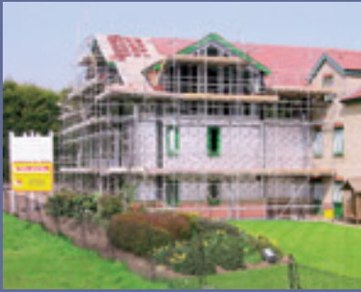
Works progressing on the Bentley Hotel
