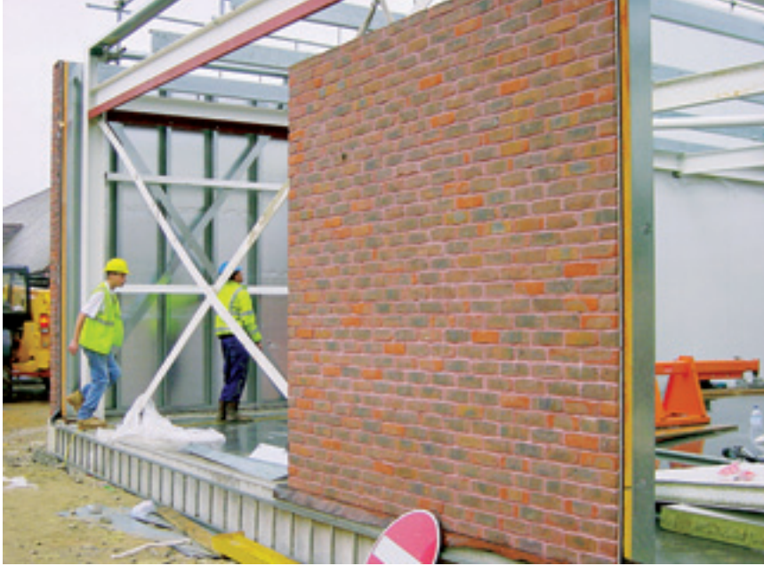
Cladding panel being fitted on site
