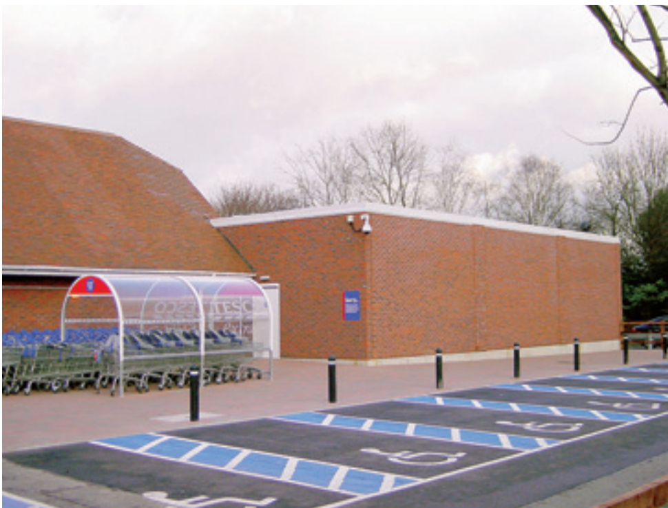
The cladding system in use on a Tesco superstore extension
