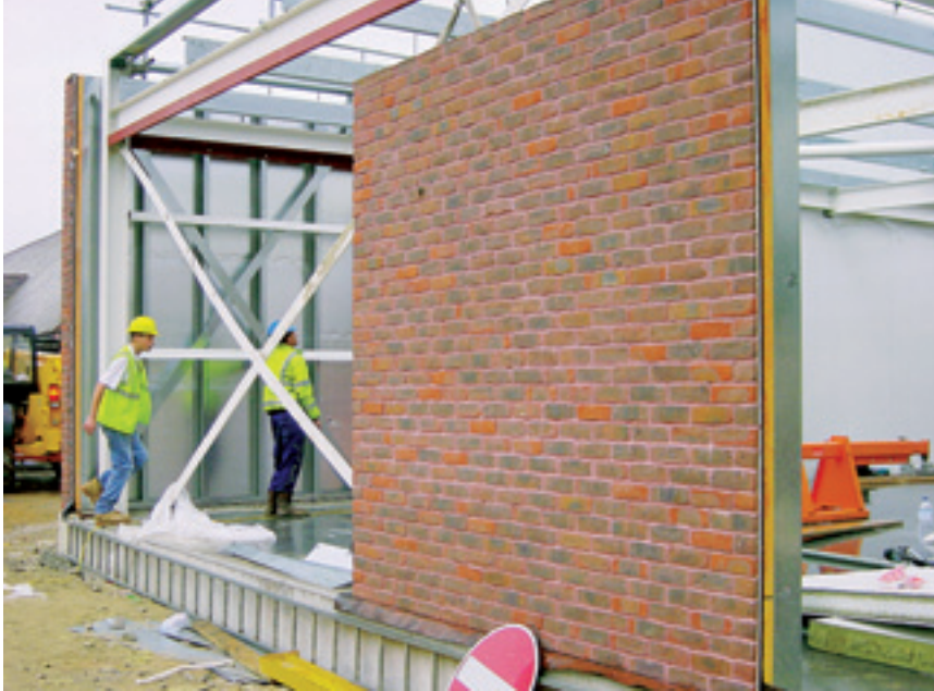
Cladding panel being fitted on site
