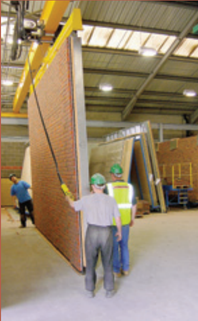
A completed cladding panel being stored at the factory
