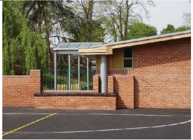
Rainwater collection downpipe and a lift-up seat incorporating an in-line filter
