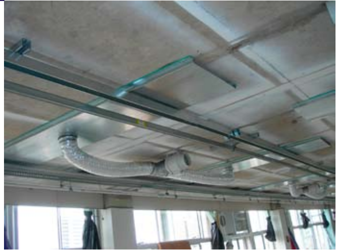
CoolDeck being installed
